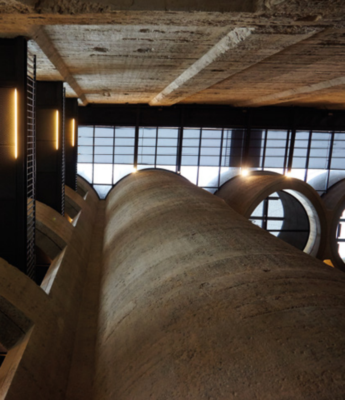
VANTAGE POINT Interesting angles provide a different perspective of the architectural feat achieved with the reimagining of the Zeitz MOCAA building.
