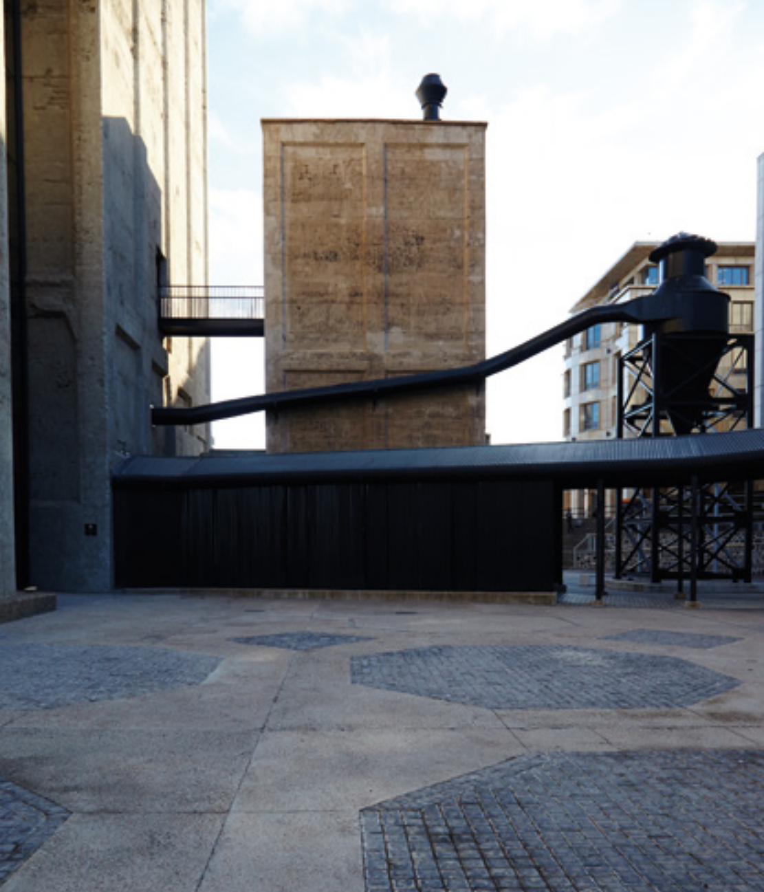
MULTI-FUNCTIONAL Once used to deliver grain from the shipping elevator to the shiploaders, the gantry has been transformed into a coffee shop.
